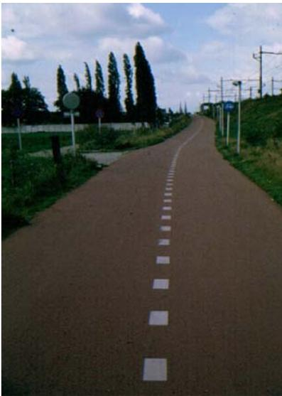
Finally, this scene shows a good feature that is common on paths abroad but rare in Britain – the centre line. Discipline on cycle paths is poor and head-on collisions between cyclists have resulted in death and serious injury. Centre lines are needed every bit as much on cycle paths as on roads, as are other frequent reminders to keep left.
