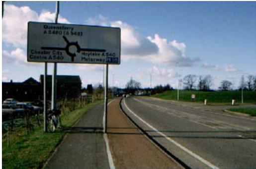
A cyclist was badly hurt riding into this sign support, barely visible at dusk. No-one would build a road without adequate clearances, but for some reason it is acceptable to place structures, and dark ones at that, right up to or even within a path for cyclists.
