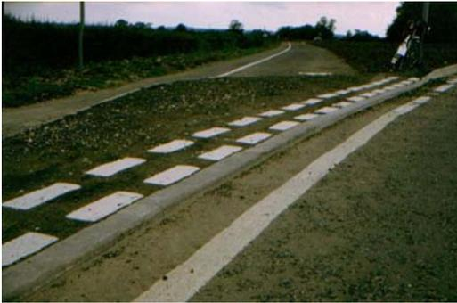
A common gripe with cyclists is poor surfaces and upstands. Cycle paths should *not* end with dropped kerbs, but should arrive at road level and there should be a perfectly flush join back from the junction itself. Again this is normal practice in road building and was common, too, in the cycle paths of the 1930s. Once more, there seems to be confusion between design for cyclists and design for pedestrians.
