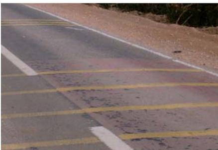
Rumble strips are not only uncomfortable but can be dangerous if encountered at even moderate speed. The advice to leave at least a 0.75m gap to each side for cyclists is rarely heeded.
